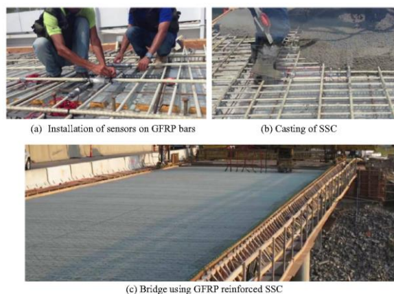
Figure 2. Demonstration project with SWSSC
