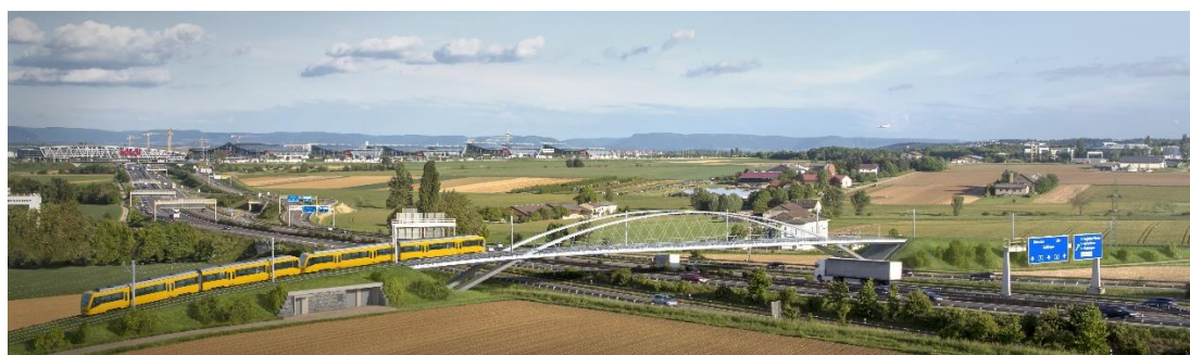
Figure 3. Network arch bridge designed by Schlaich Bergermann Partner for the City Public Transport Operator Stuttgarter Straßenbahnen (SSB) fully suspended on CFRP hangers. Length of the network arch: 80 metre. Source of rendering: Stuttgarter Straßenbahnen AG.
